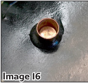
Image 16: End Cap set in epoxy on back of glass
